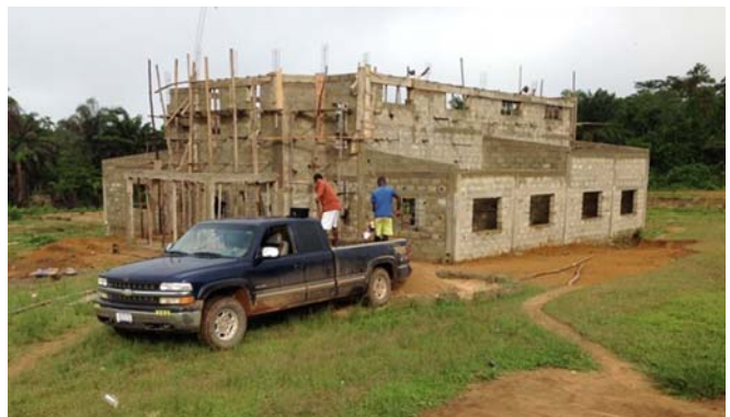
Church construction, Morweh School, Liberia, Africa
